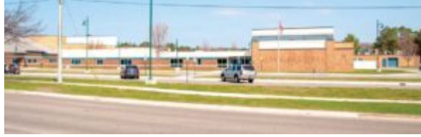
The current Shay Elementary School will be demolished and a new K-4 elementary school will be built as part of the $41.85 million bond project voters approved last week. (Harbor Light Newspaper photo/Mark Flemming)
